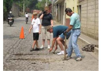
“We only did half of three [speed bumps] today. We basically clear the stone and concrete. The stones are easy, use a chisel and hammer. The concrete, you dig under it and break it with a big hammer or use a huge steel pick and get leverage under it.”
