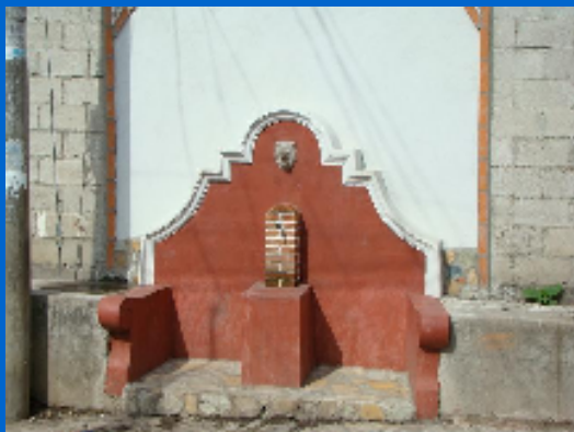
One of 10 water fountains that have been completed
