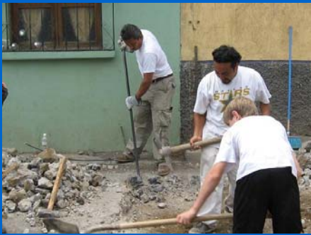
Speed bump construction
