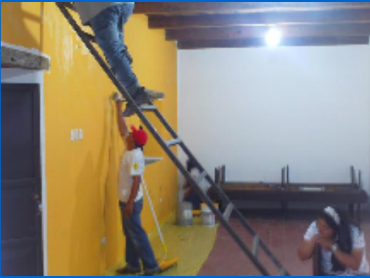
Painting the inside of the San Pedro city hall.
