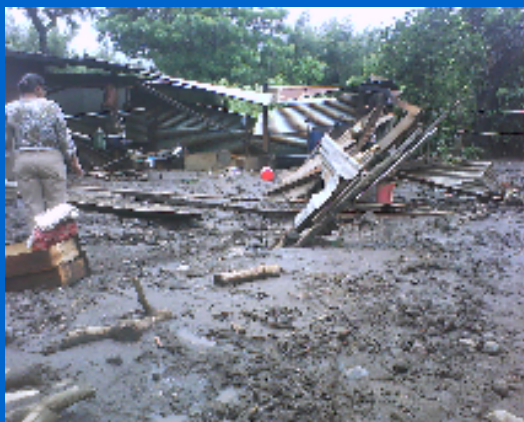
Remains of a destroyed home.
